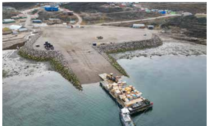
Kinngait's new sealift ramp and laydown area
