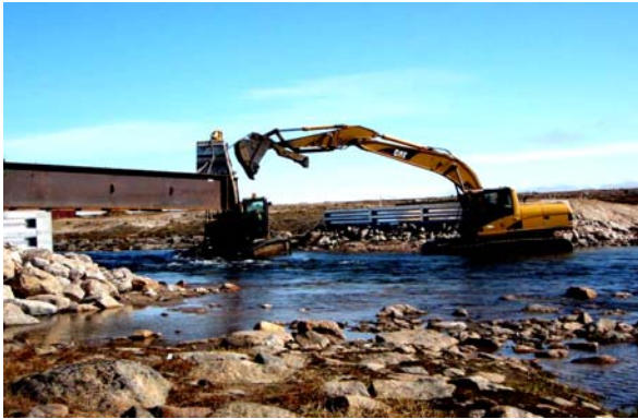
Figure 1: Pulling the Structure across the River
