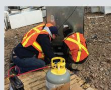
• Remove compressor and drain mineral oil • Remove refrigerant
